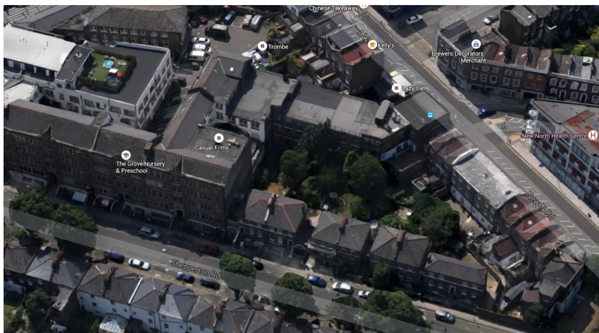
Image 2: Aerial View of the site from the north.
